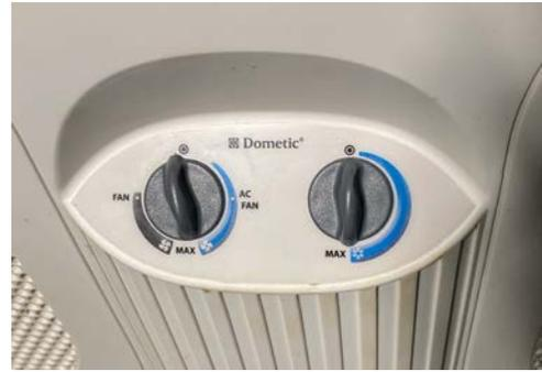
These buttons are on the lower left of the MAGNUM battery monitor above the sink. Turn the AC knob on the left clockwise to Max AC and the other one to max cooling. If running AC overnight you will want to turn the left knob to the low AC/FAN setting and the temperature setting to about 2/3 the way up. If using the generator, you can turn the charger back on after the AC starts.
